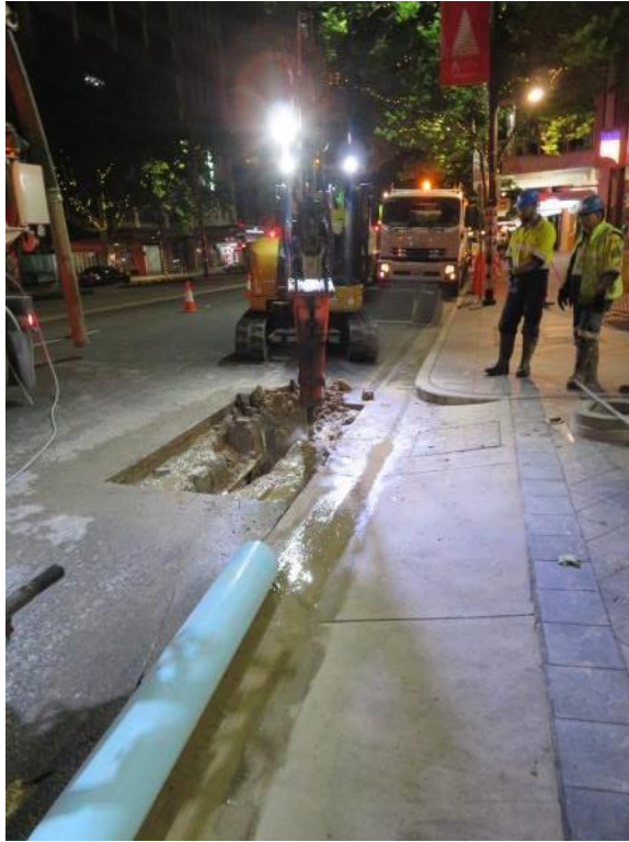
Proactive night repair King William
