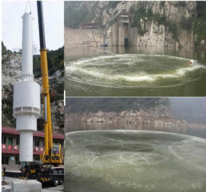
Water-lifting aerators and its application in Heihe Reservoir
