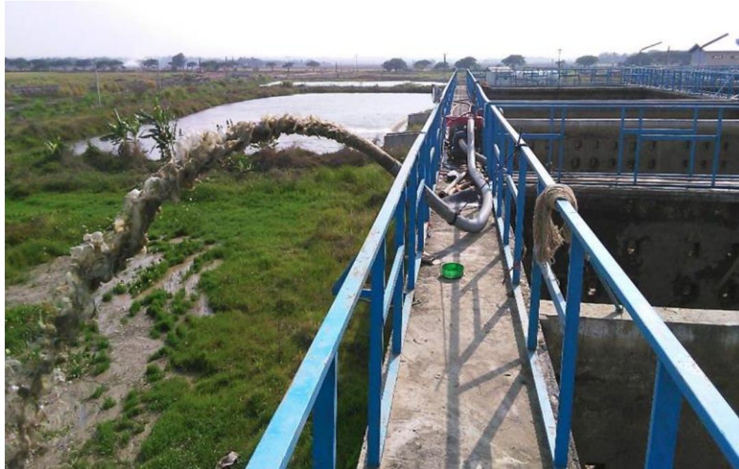
Discharging sludge from the sedimentation tanks
