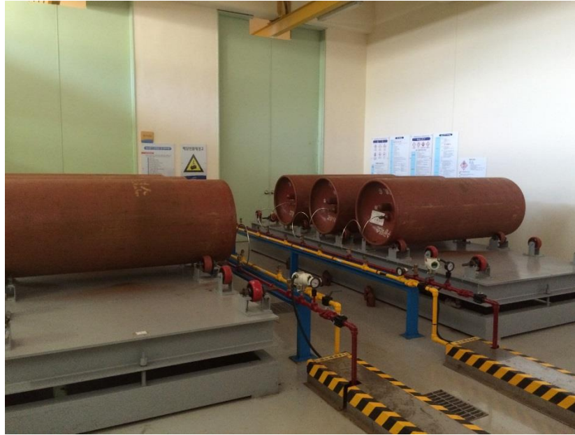
Chlorine Storage Tank (left) and Feeding System (right)
