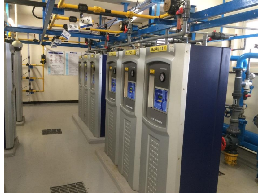
Chlorine Storage Tank (left) and Feeding System (right)
