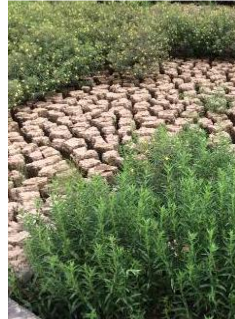
Sludge drying bed
