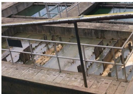
Figure 4a Baffled channel flocculator
