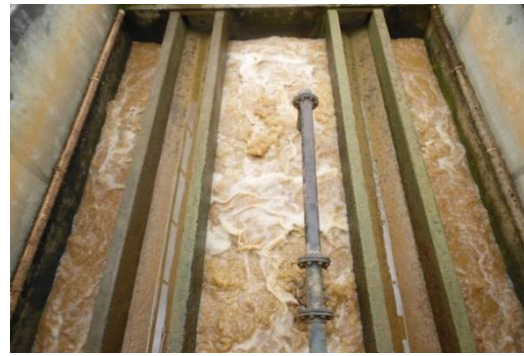
Figure 7b Filter Backwashing
