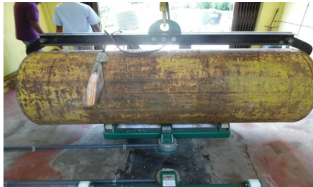
Figure 6 Gas chlorine cylinder on weighing gauge
