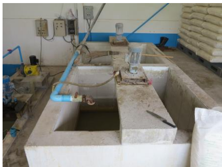
Figure 2 Alum Solution Tank
