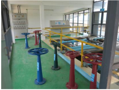
Figure 19 Identification of valve color
