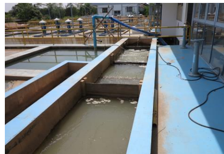
Figure 7 Hydraulic Mixing (1 basin)
