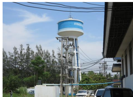
Figure 11 Elevated Tank for Backwashing (120 m 3 )
