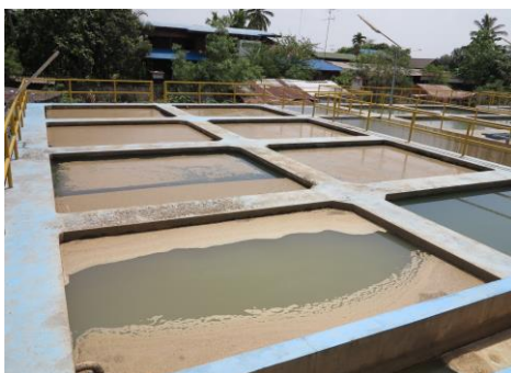
Figure 15 Scum in Sedimentation Basin
