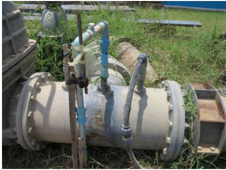
Figure 4 Static Mixer (Alum)
