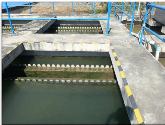
Figure 6 Sedimentation (2 basins)
