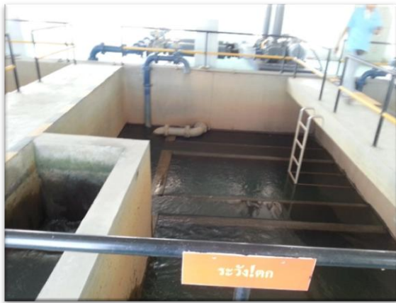
Figure 8 Filtration (4 basins)
