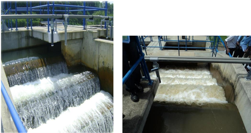
Figure 4 Cascade aerator
