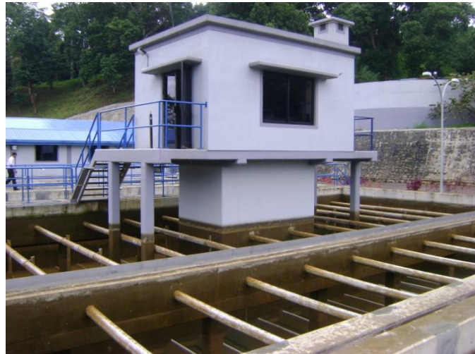
Figure 5 Pulsator clarifier
