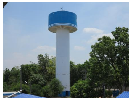
Figure 10 Elevated Tank for Backwashing (500 m 3 )
