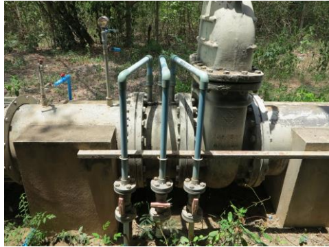
Figure 4 Static Mixer (alum and chlorine)
