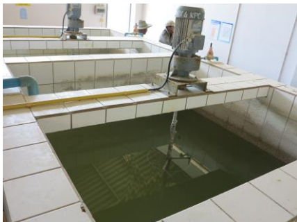
Figure 2 Alum Solution Tank
