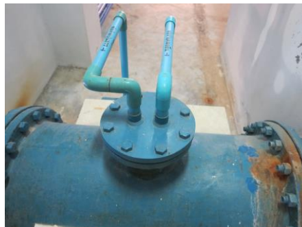
Figure 17 Lime injection pipe
