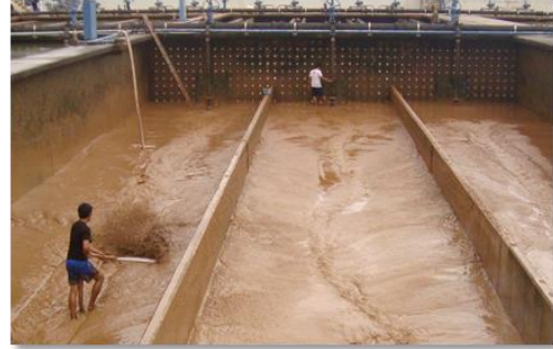
Figure 9 Sedimentation Tank (4 basins) and Manual Cleaning in Chinaimo WTP
