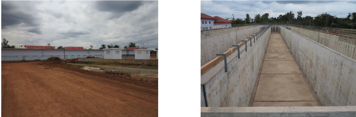
Figure 14 New water treatment plant under construction
