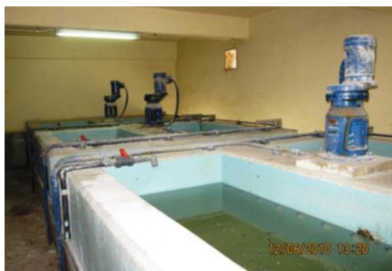
Figure 2 Alum Solution Tank
