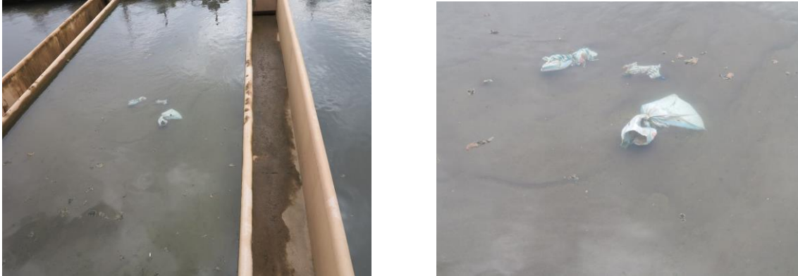
Figure 12 Filter basin of Chinaimo WTP
