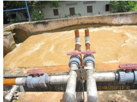
Figure 6 Hydraulic Jump (pre chlorine)
