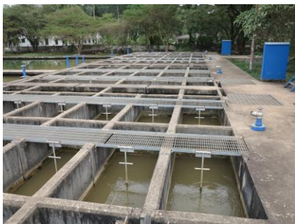
Figure 7 Vertical baffle channel (8 basins)
