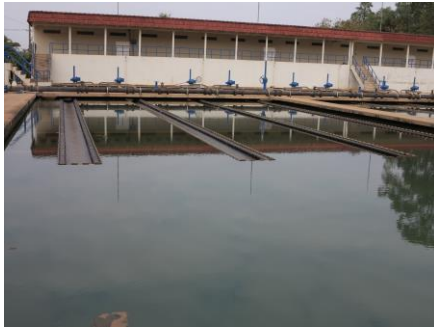
Figure 9 Sedimentation Tank (4 basins) and Manual Cleaning in Chinaimo WTP
