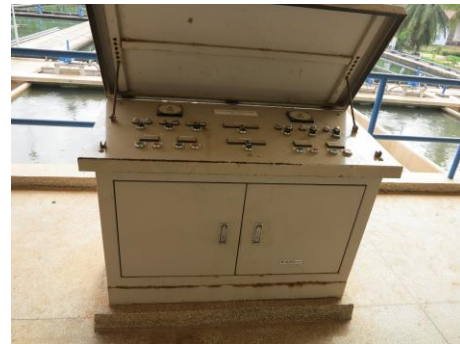
Figure 10 Filter Tank (8 basins) and Backwash Control Panel
