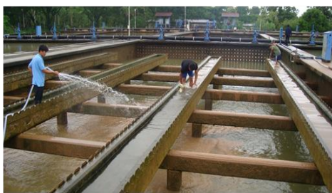
Figure 11 Sedimentation cleaning of Chinaimo WTP
