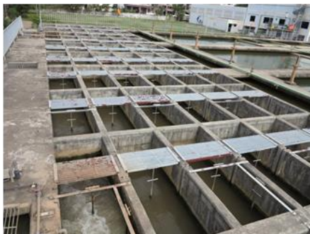
Figure 7 Vertical Baffle Channel (8 basins)
