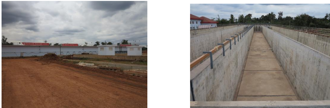
Figure 15 New Plant under Construction
