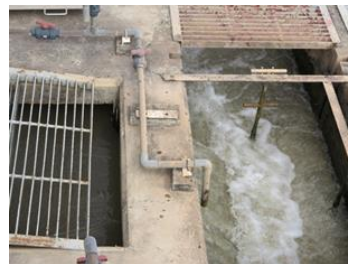
Figure 5 Polymer injection site
