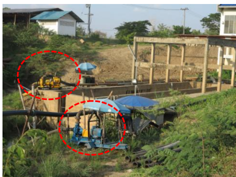
(c) Additional pumping equipment installed
