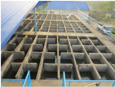
Figure 6 Baffle Channel Type
