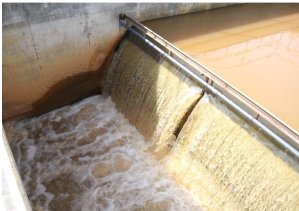
Figure 8 Rapid Mixing Elevated Chamber
