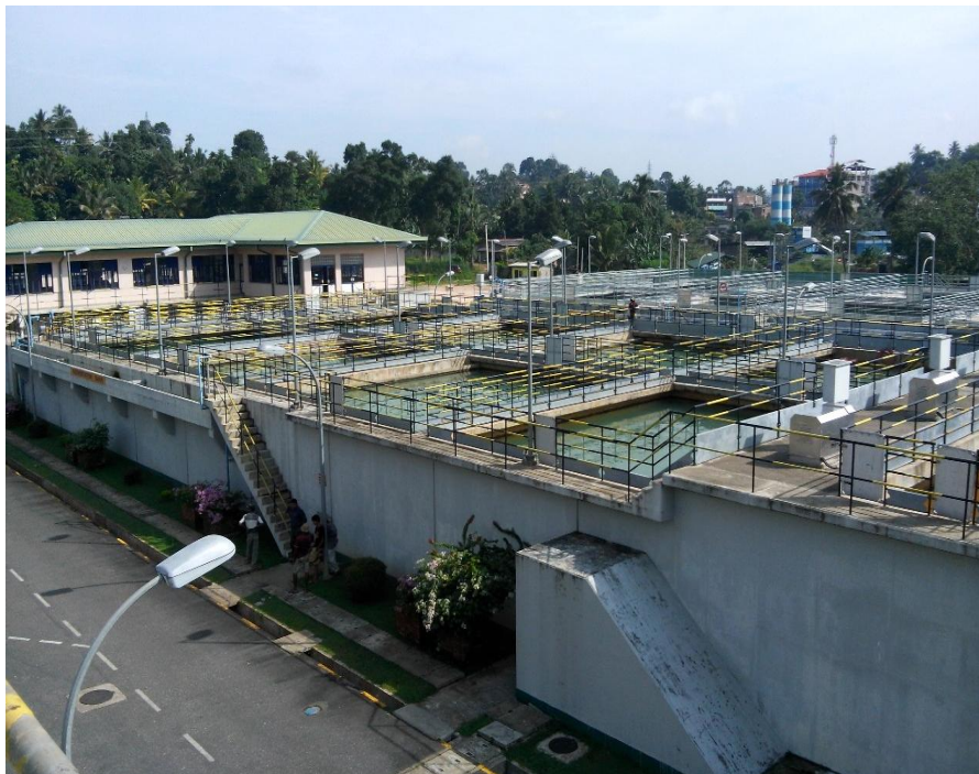
Figure 1 Greater Kandy Water Treatment Plant
