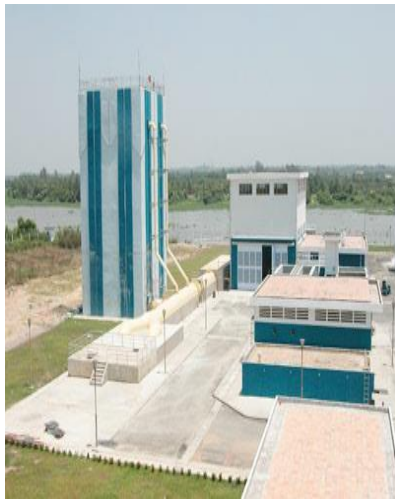
Figure 2 Hoa Phu Raw Water Pumping Station
