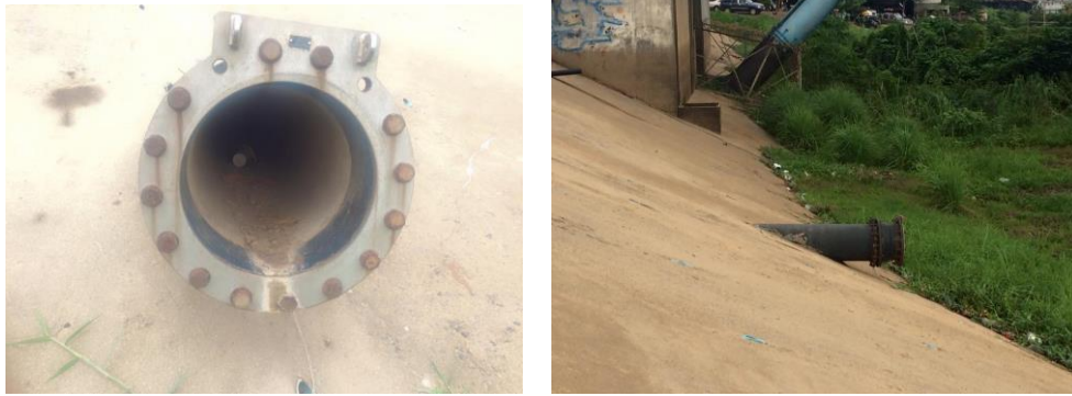
Figure 9 Sludge outlet at the down stream of the river
