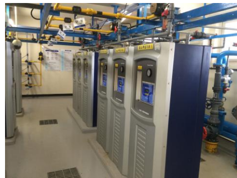
Figure 4 Chlorine Storage Tank (left) and Feeding System (right)
