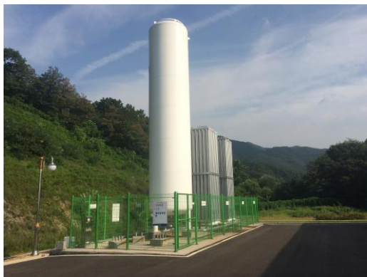
Figure 2 Carbon Dioxide Storage Tank (left) and Powdered Activated Carbon Feeding System (right)
