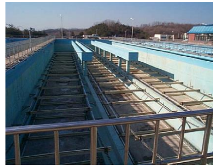
Figure 9 Chain-and-Flight Type Collector
