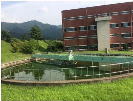
Figure 11 Gravity Thickener
