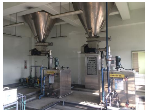
Figure 2 Carbon Dioxide Storage Tank (left) and Powdered Activated Carbon Feeding System (right)
