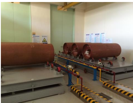
Figure 4 Chlorine Storage Tank (left) and Feeding System (right)
