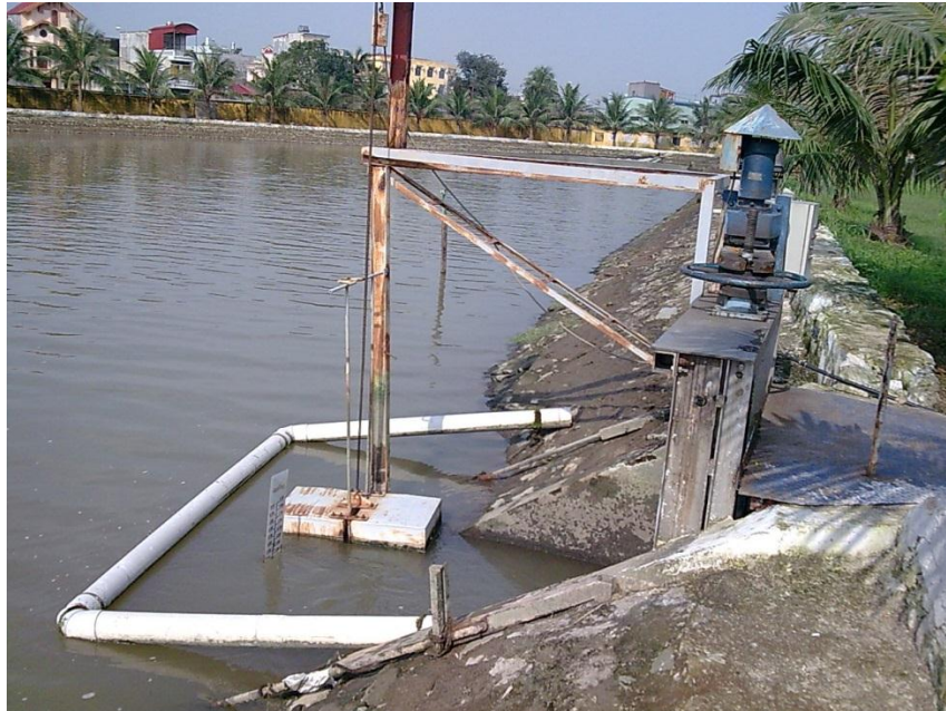
Figure 4 Pre-sedimentation Tank of An Duong Water Treatment Plant
