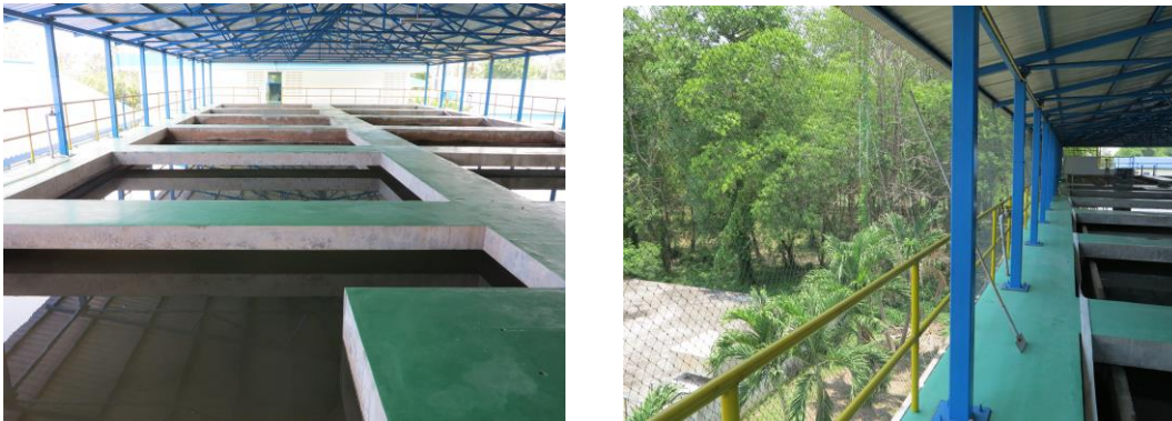
Figure 16 The roof (left) and net (right) of flocculation and sedimentation basin building
