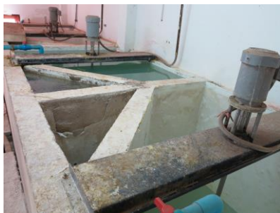
Figure 2 Alum (Solid) Solution Tank (left) and Chlorine ( \text{CaOCl}_2 ) Solution Tank (right)
