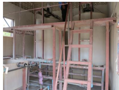
Figure 2 Alum (Solid) Solution Tank (left) and Chlorine ( \text{CaOCl}_2 ) Solution Tank (right)
