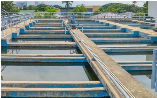
Figure 6. Super Pulsator Clarifier
