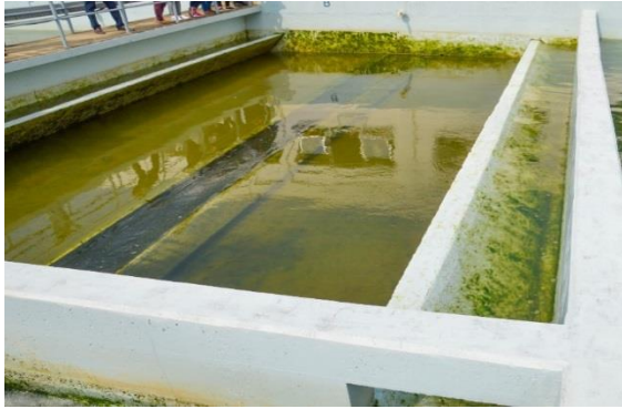
Figure 7 Rapid sand filter (9 basins)
