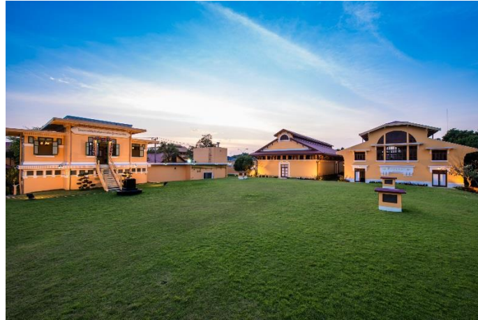
Figure 23 Thai Waterwork Museum at Samsen WTP
