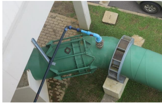
Figure 5 Alum injection
