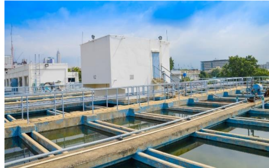
Figure 6. Super Pulsator Clarifier
