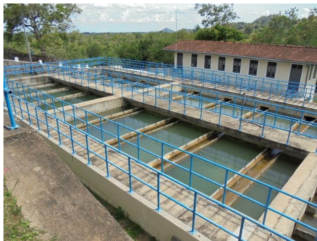
Figure-5: Sedimentation basin
