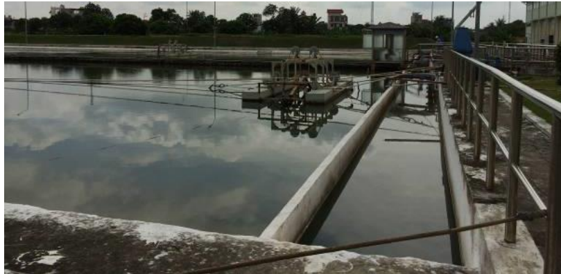
Figure 6 Horizontal sedimentation tank
