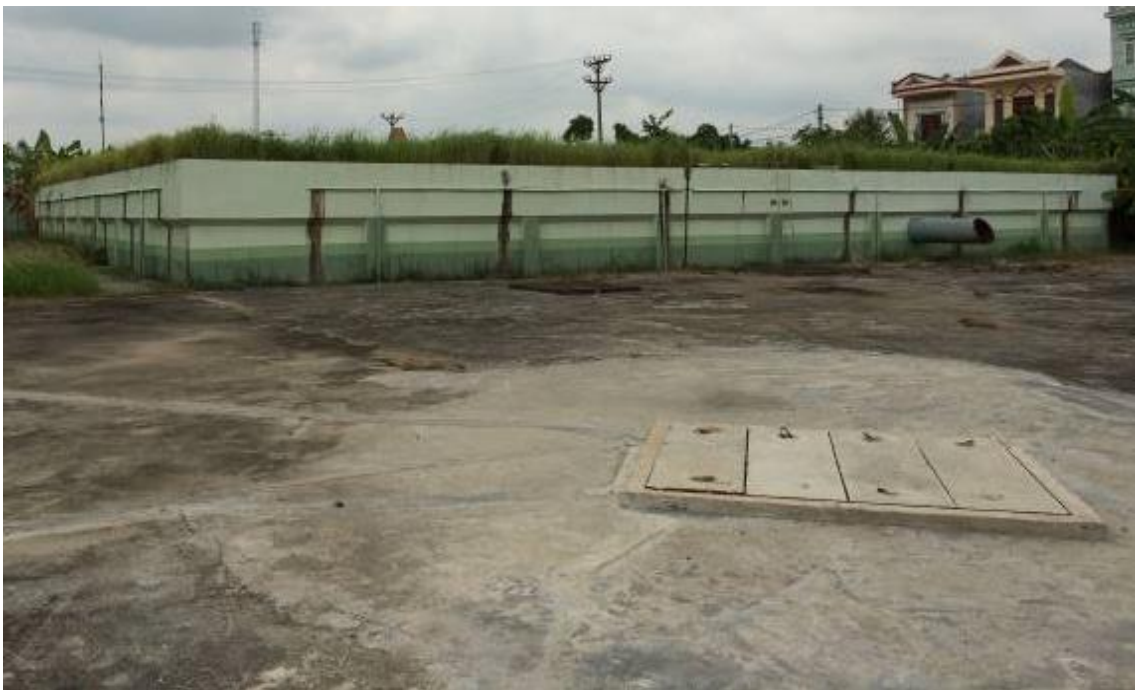
Figure 10 Purified water storage tank
