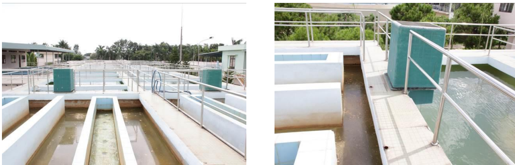
Figure 4 Chemical reaction tank
