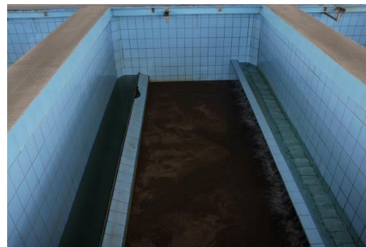
Figure 7 Rapid filtration tank
