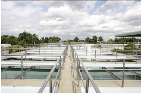
Figure 5 Sedimentation tank and weir system
