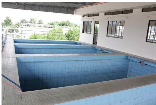
Figure 7 Rapid filtration tank
