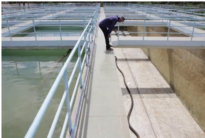
Figure 6 Maintaining of sedimentation tank
