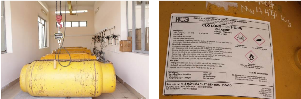
Figure 18 Chlorine tank
