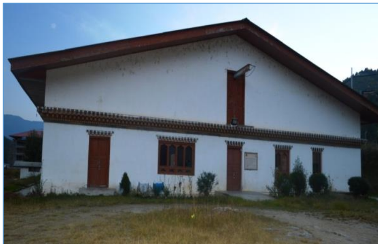
Figure 1: Jungzhina Water Treatment Plant
