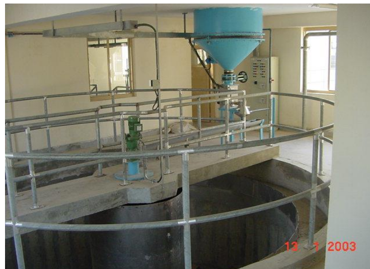
Figure 8: Lime Dosing
