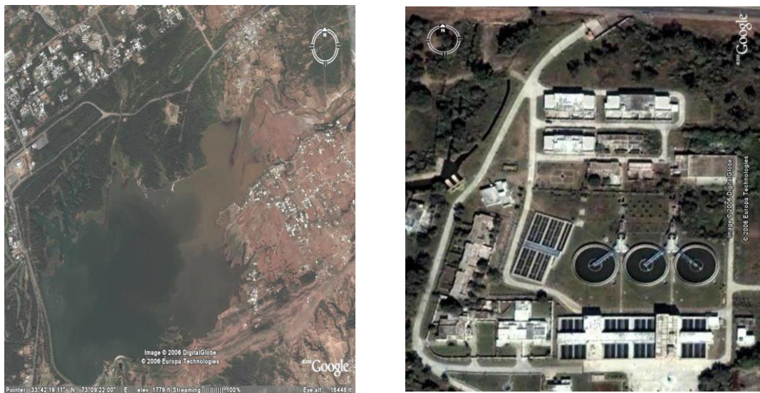
Figure 1: Rawal Lake Source (Left) and Rawal Lake Water Treatment Plant (Right)
