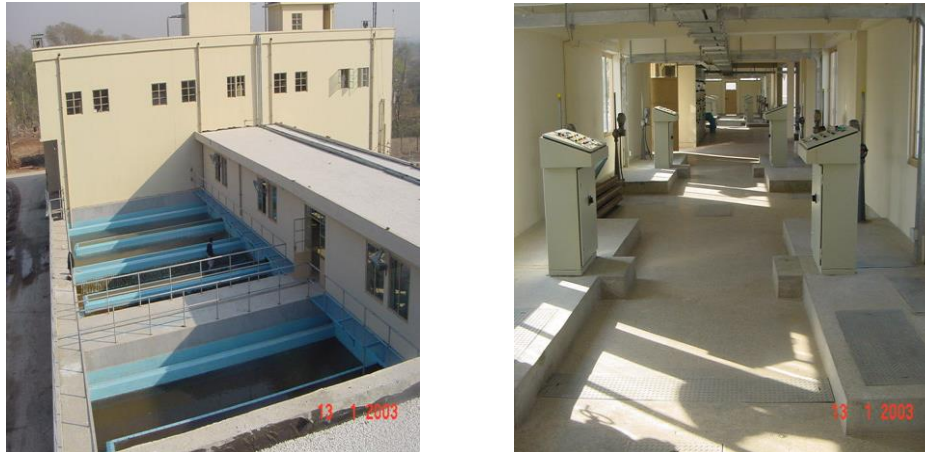
Figure 7: Rapid Sand Filtration
