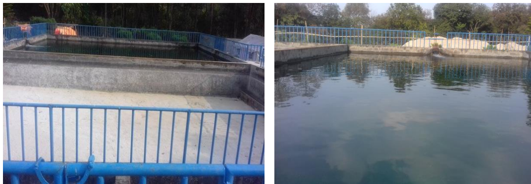
Figure 4: Slow Sand Filter
