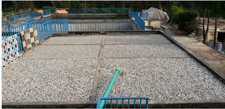
Figure 3: Horizontal Roughening Filter
