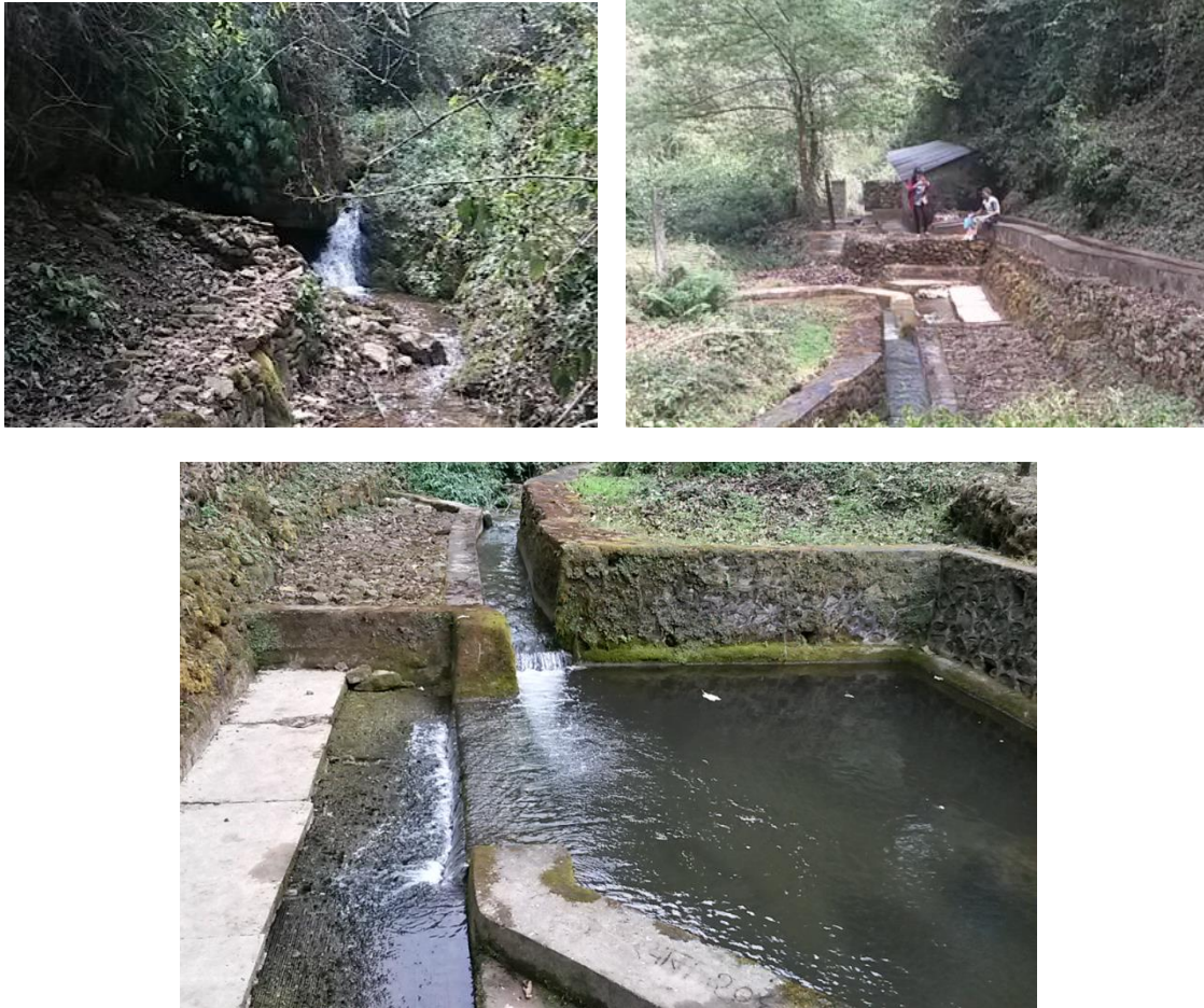
Figure 2: Intake works of DWTP at the Khar Stream
