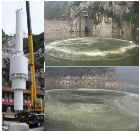
Figure 23 Water-lifting aerators and its application in Heihe Reservoir
