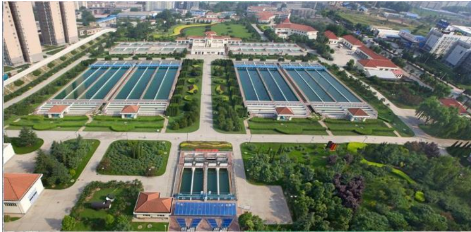
Figure 3 Water treatment unit at XSWTP
