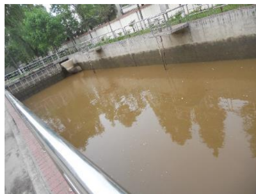
Figure 17 Wasted sludge equalization tank
