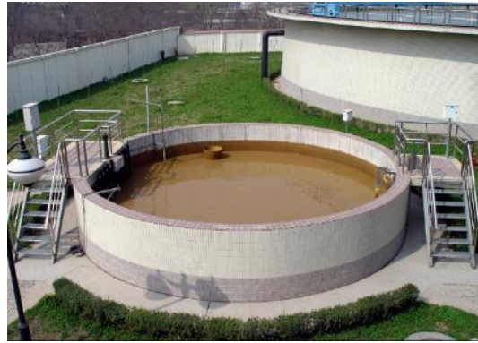
Figure 19 Thickened sludge storage tank
