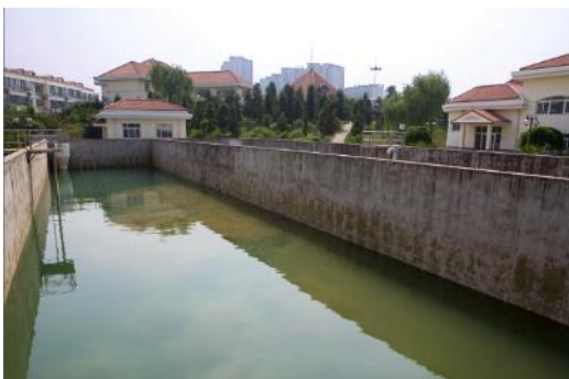
Figure 16 Reuse water equalization tank
