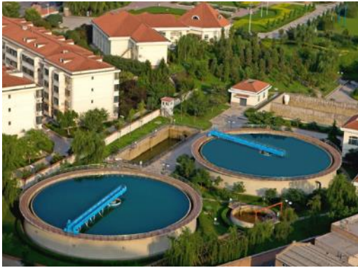
Figure 18 Sludge thickening tank
