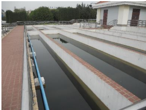
Figure 12 Vertical flow folded-plate flocculating tank
