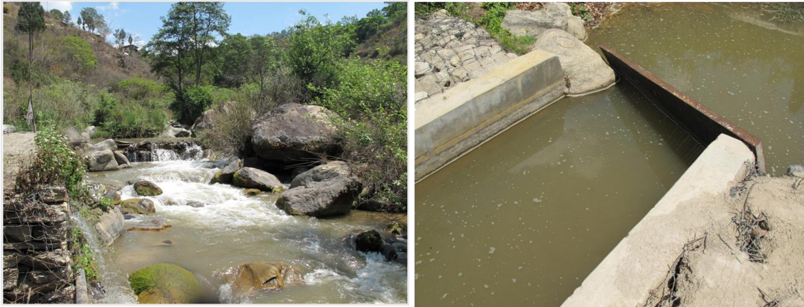
Figure 1 Baychu Source and intake
