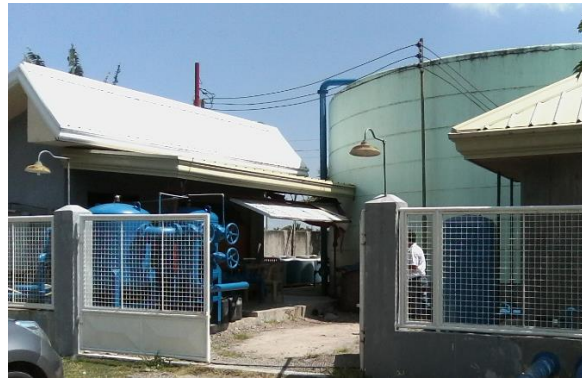
Figure 7 SFVR Pumping Station
