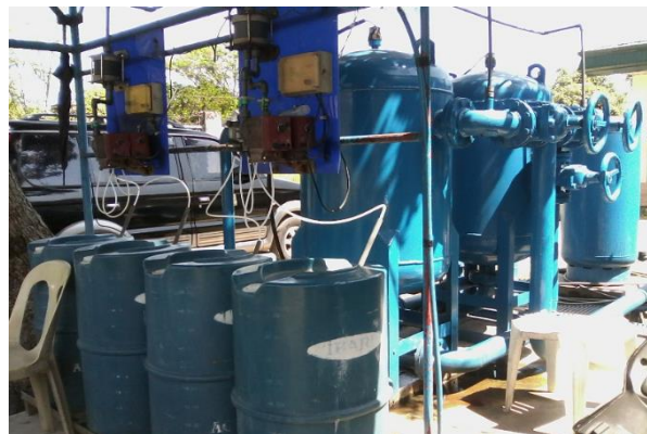
Figure 4 Fortuna Pumping Station
