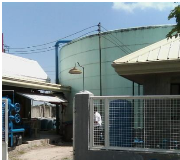
Figure 14 Water Reservoir at SFVR Pumping Station
