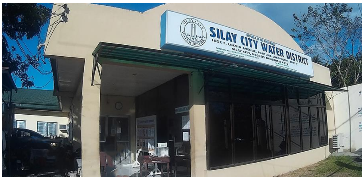
Figure 1 Office of Silay City Water Distirct
