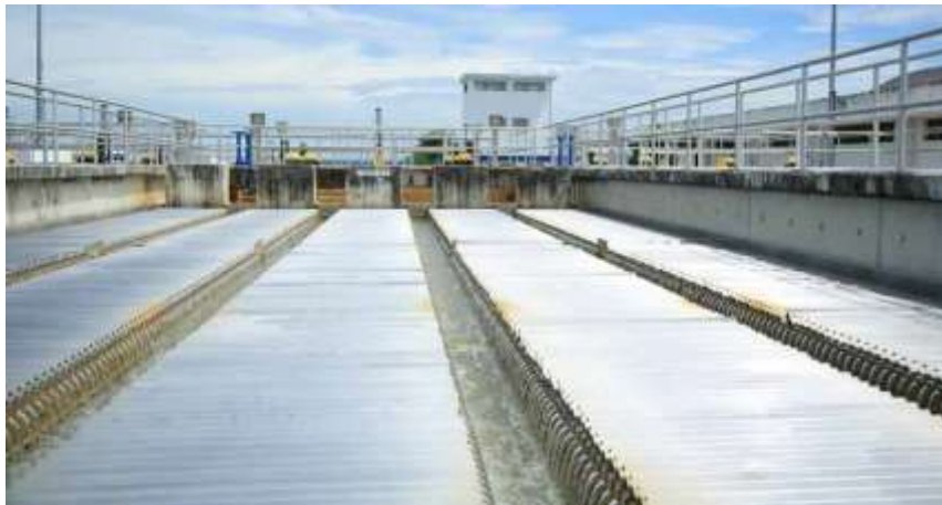
Figure 11: Multi-tray Sedimentation Tank
