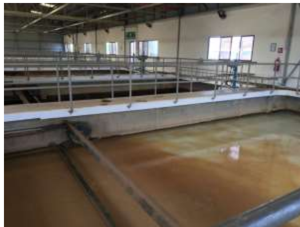
Figure 12: Dissolved Air Floatation Units
