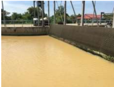
Figure 6: Bar Screens at the inlet of the Balancing Pond
