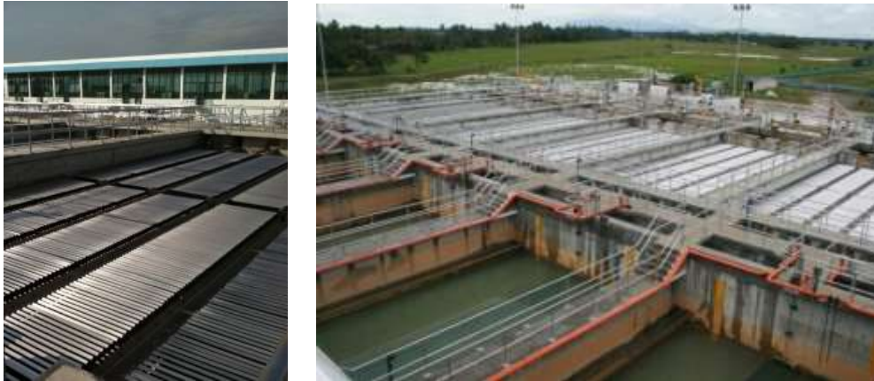
Figure 13: Lamella clarifier with inclined stainless steel plates
