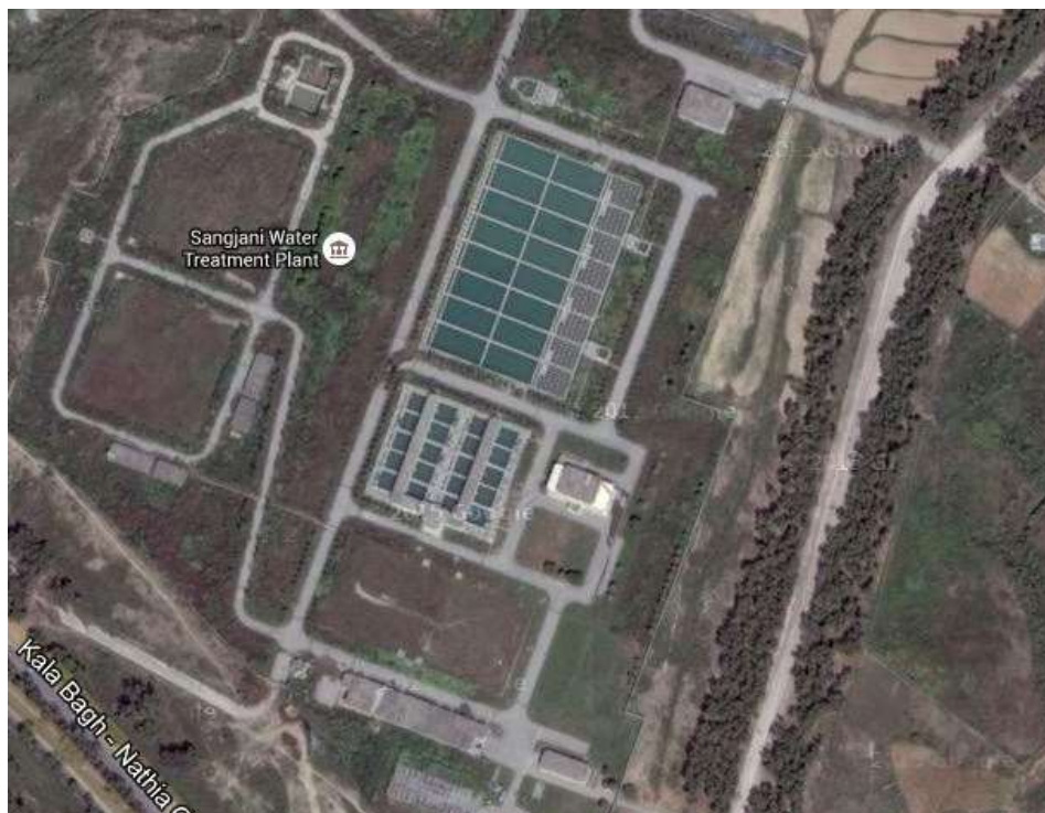
Figure 1: Sang-Jani Water Treatment Plant
