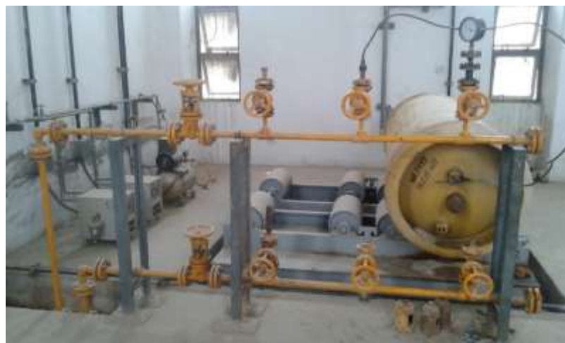
Figure 9: Chlorinator
