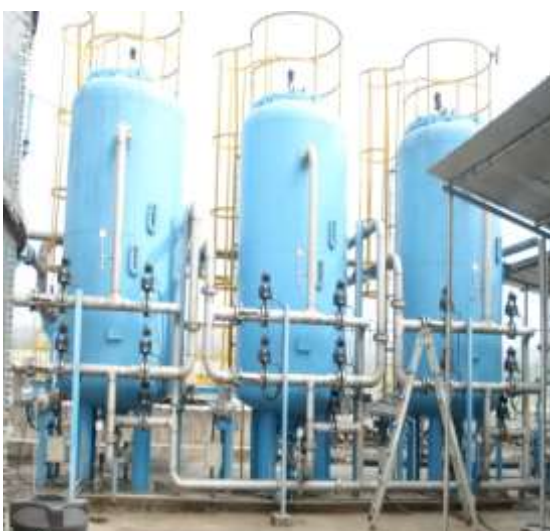
Figure 4 Pressure filters
