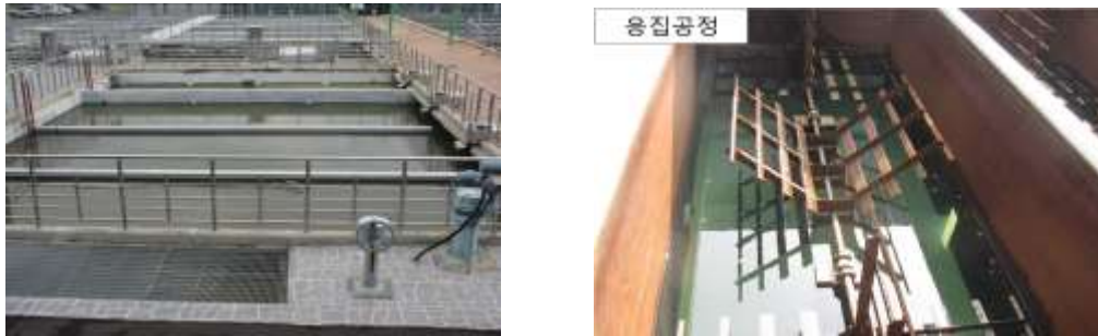
Figure 5 Horizontal shaft with paddle flocculator (4 basins)
