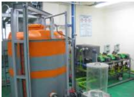
Figure 2 Coagulant storage tank (left) and feed system (right)
