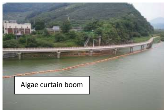
Figure 13 Algae curtain boom of Nakdong River (water intake)
