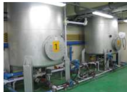
Figure 3 Chlorine storage tank (left) and lime feed system (right)
