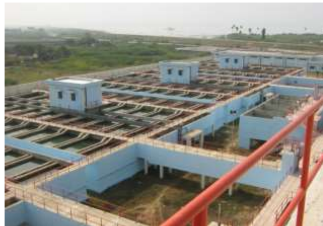
Figure 4. Pulsator clarifier
