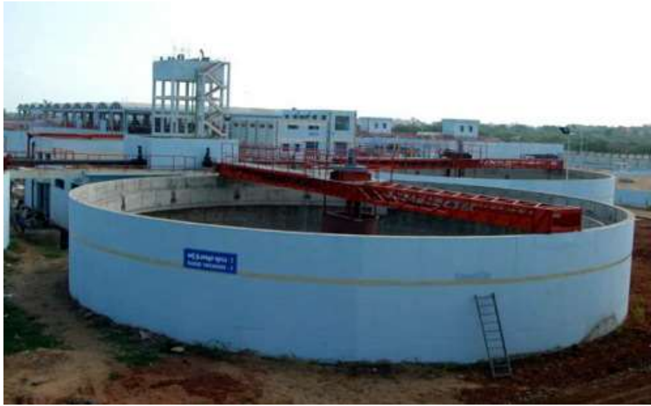
Figure 12. Sludge Thickener
