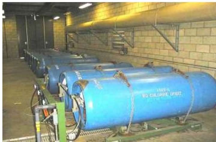
Figure 2. Chlorine containers
