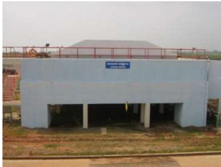
Figure 3. Cascade aerator
