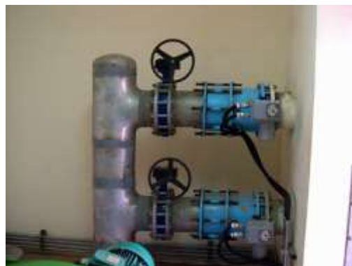
Figure 6. Vacuum break valve
