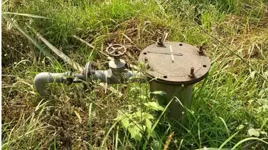
Figure 3: Bore holes inside the water treatment facility
