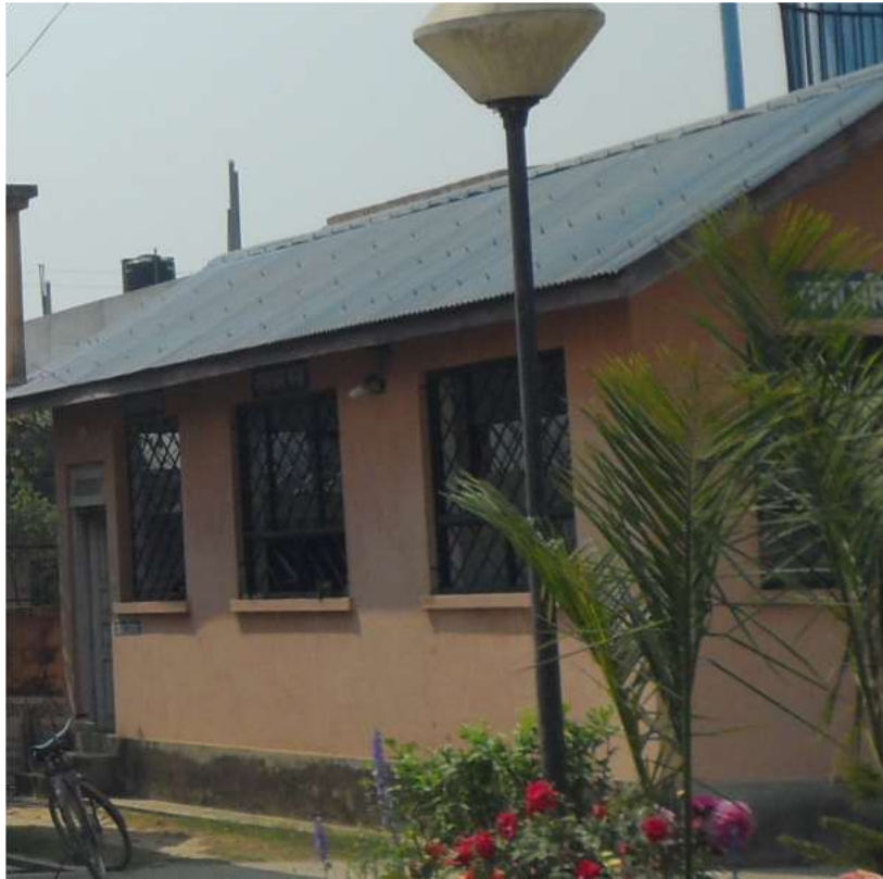
Figure 4: Facility for the storage of chemicals
