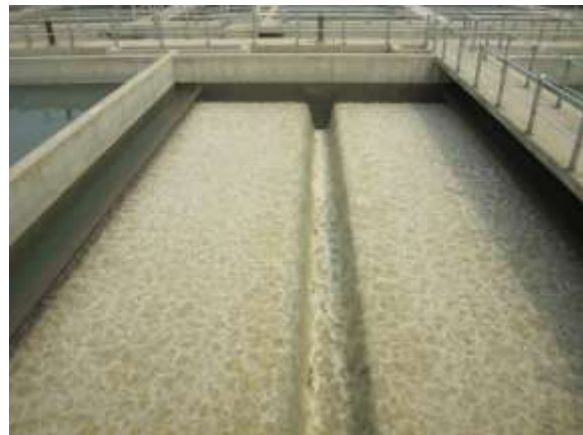
Figure 7: Filter units during filtration (left) and during backwashing (right)
