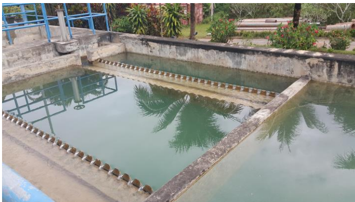
Figure 11 Filter Tank (4 basins) and arrangement of materials in the filtration unit
