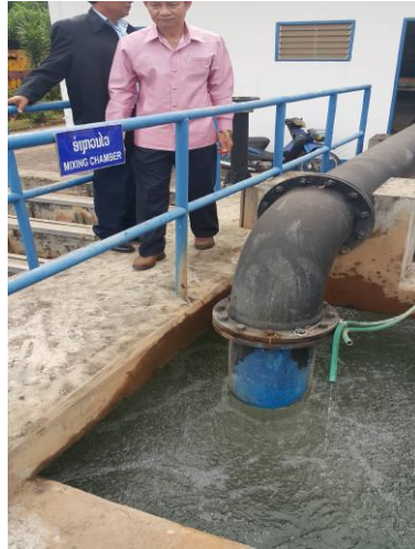
Figure 7 Static Mixer (Alum)
