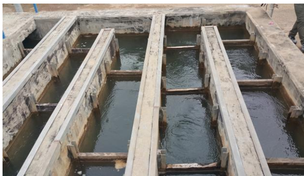
Figure 8 Vertical baffle channel
