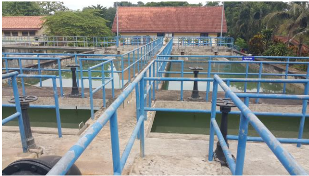
Figure 10 Sedimentation Tank (4 basins)(left) and a schematic diagram of the tank (right)
