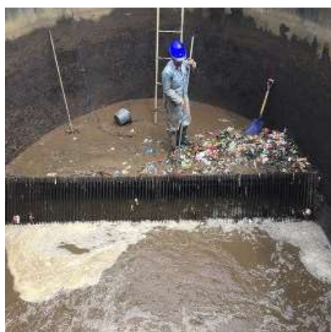
Figure 4 Cleaning at the Cikapundung river water intake Source: PDAM Tirtawening twitter
