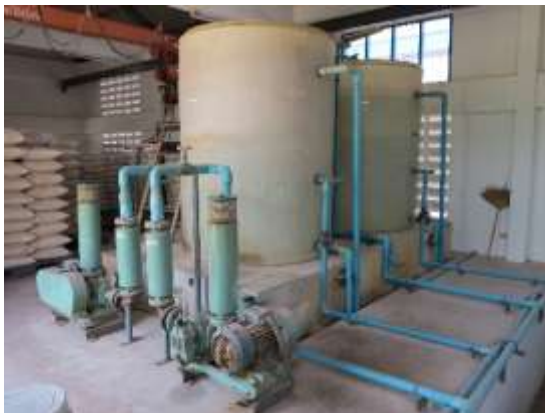
Figure 2 Alum solution tank (left) and storage tank (right)
