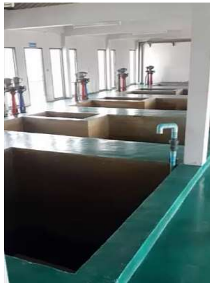
Figure 8 Filter Tanks
