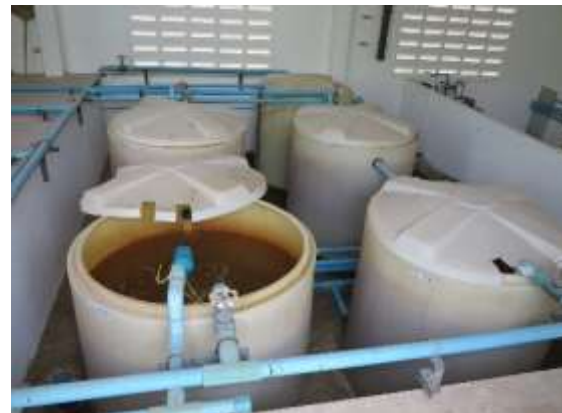
Figure 2 Alum solution tank (left) and storage tank (right)
