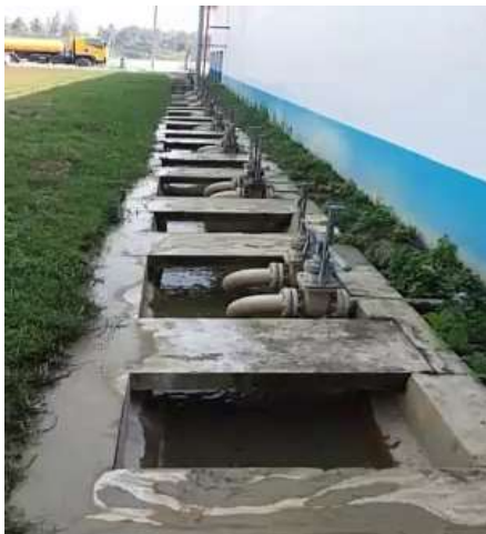
Figure 11 Sludge canal
