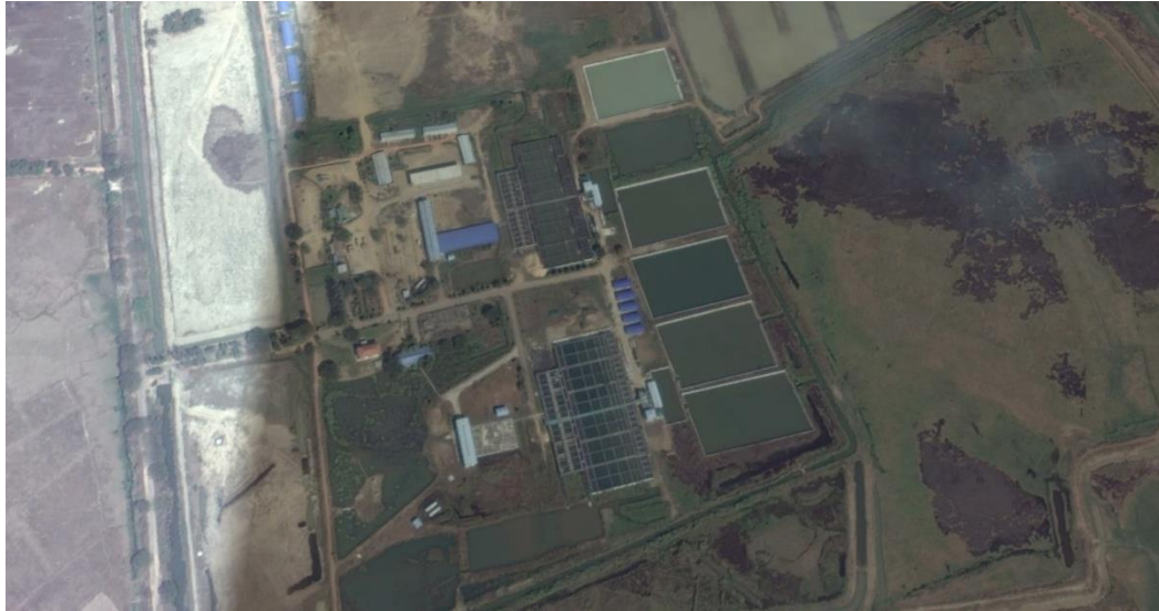
Figure 2: Aerial view of Nyaungnapin WTP
