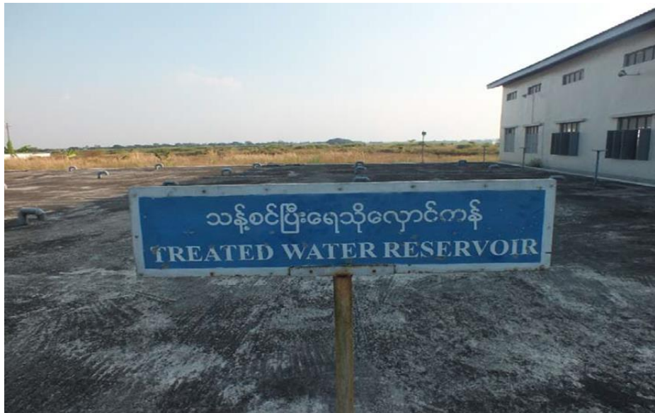
Figure 15: Clear Water Well (or Treated Water Storage Tank)
