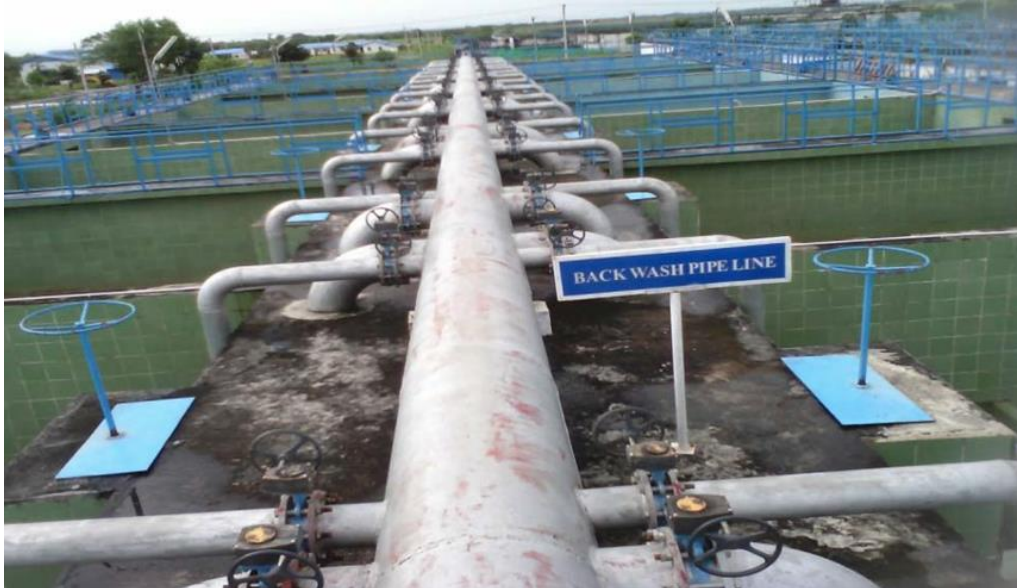
Figure 14: Backwashing pipelines
