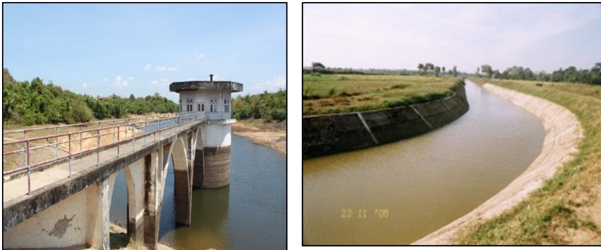
Figure 4: Nga Moe Yeik reservoir and open channel for transmission
