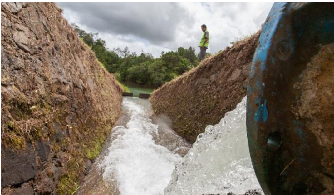
Figure 3: Under construction site of water distribution (ADB, 2015)
