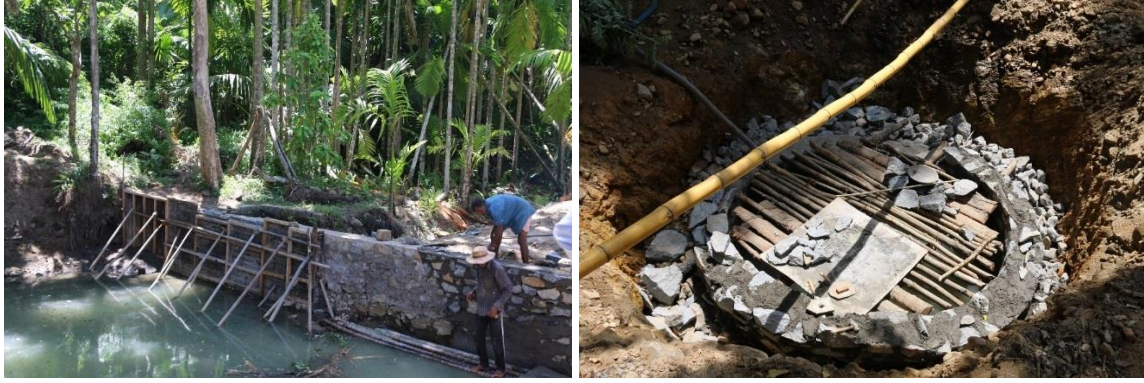
Figure 5: Construction of Rideemaliyadda South Water Supply infrastructures in Badulla District
