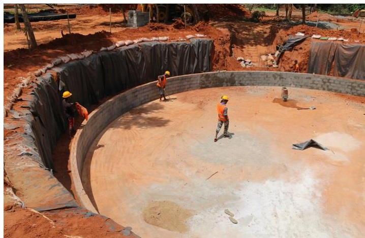
Figure 2: Construction of reservoir for Puthukudyirruppu Water Supply Plant in Mullaithivu district
