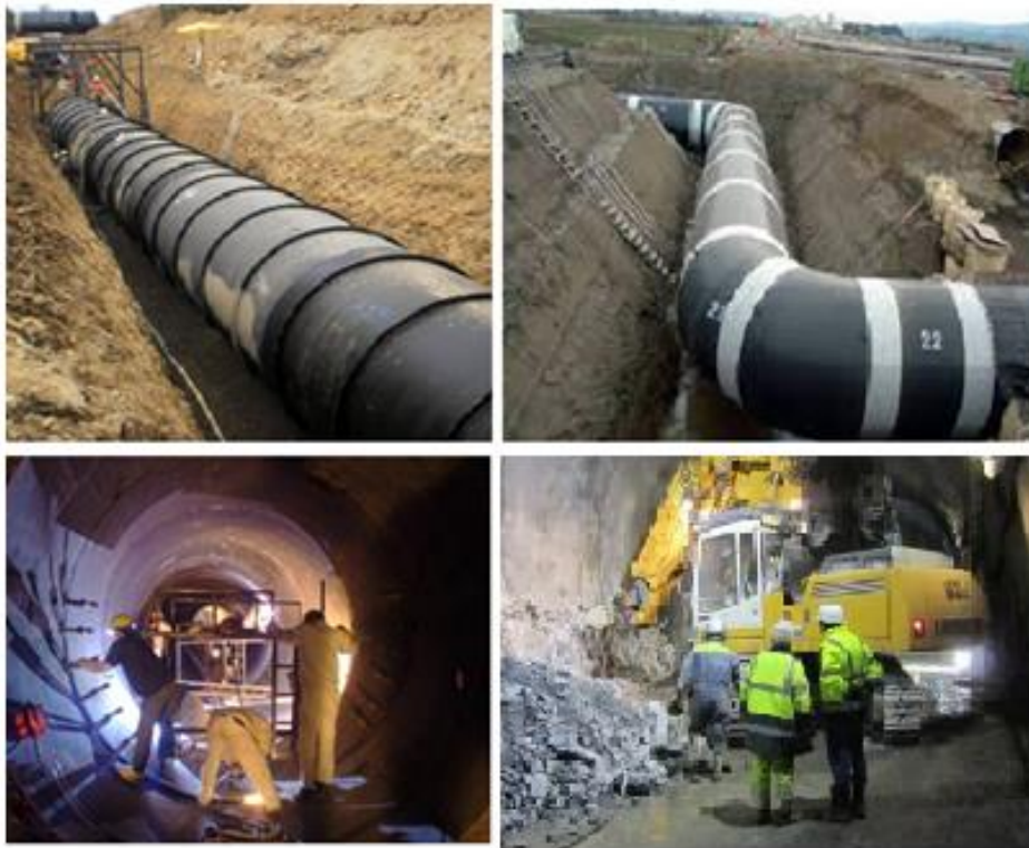
Figure 2 Construction work on the Angat Water Transmission Improvement Project (Source: mwss.gov.ph )
