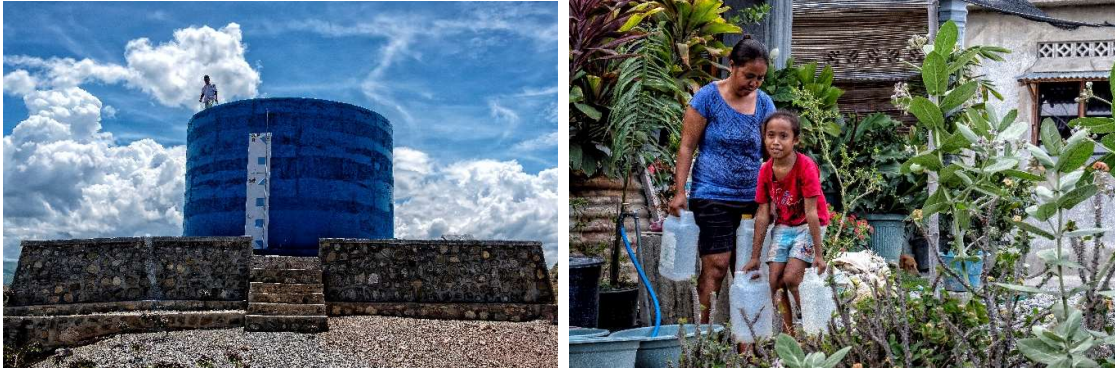
Figure 2: Water storage facilities ensured supply of safe drinking water in Timor-Leste
