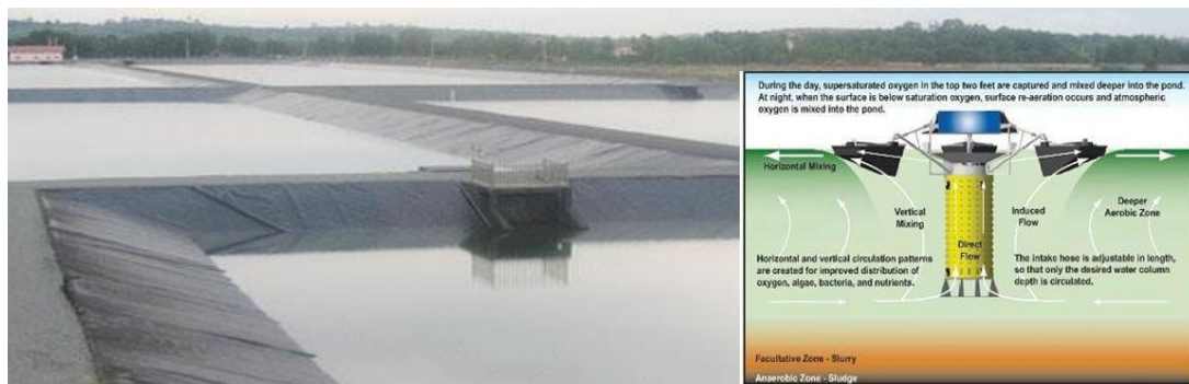
Figure 5: Existing WWTP and Proposed Solar Aerators in Sihanoukville
