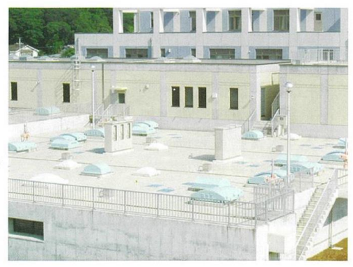
Rapid filtration basin
