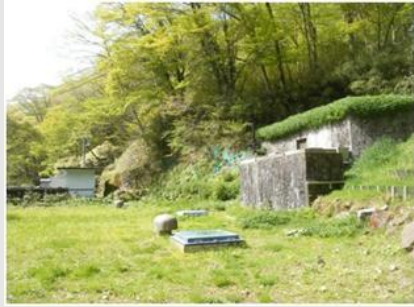
● Spring water (inside the intake facility)
