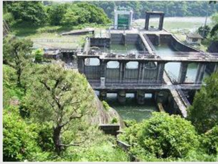
● Coagulation/sedimentation basin (rapid filtration system - horizontal)
