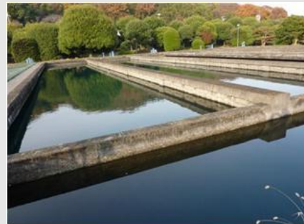
● Coagulation/sedimentation basin (rapid filtration system)
