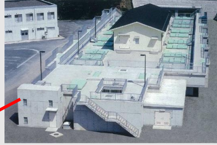
Upward Biological Contact Filtration (U-BCF)
